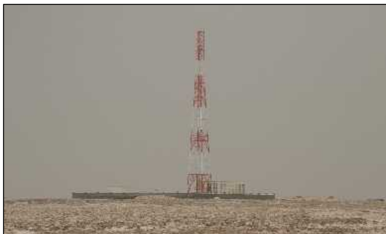
Photo: Communications tower at the Colluli site
