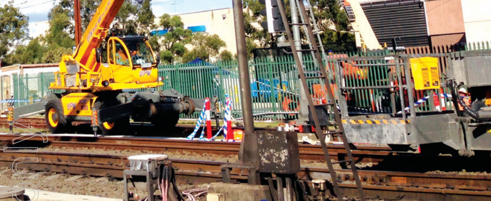
Novo Rail Alliance - Pulling HV cabling into substation, NSW.
