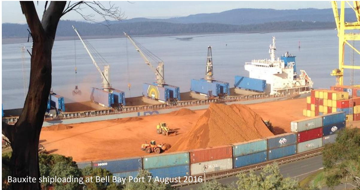
Figure 2: Bell Bay Port of Launceston can handle ships up to 65,000 tonnes. Loading is managed by QUBE Ports at more than 10,000 tonnes per day, achieving 20,000 tonnes per day during a recent loading
