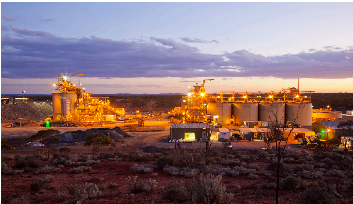
HGO Processing Plant
