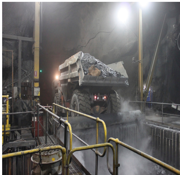
Truck Tipping at Underground Crusher
