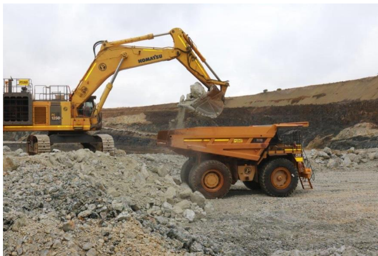
First Load In Pit
