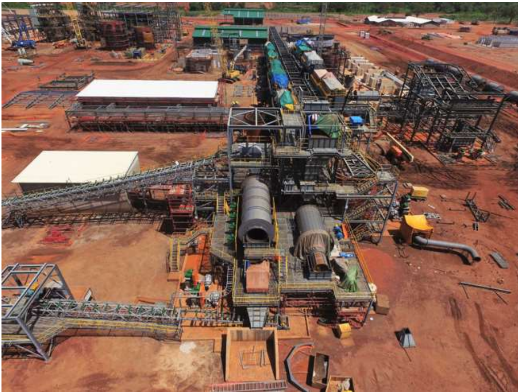
Figure 9 – Primary mill and flotation
