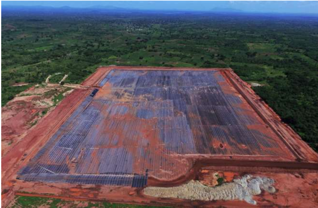
Figure 18 – Tailings Storage Facility
