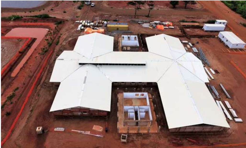
Figure 14 – Main site administration building
