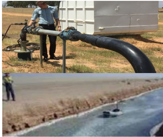
Brine Pumping from Bores and Trenches 5 Million litres successfully pumped
