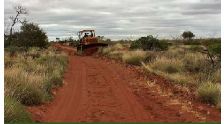
~200km of roads graded, widened or newly installed
