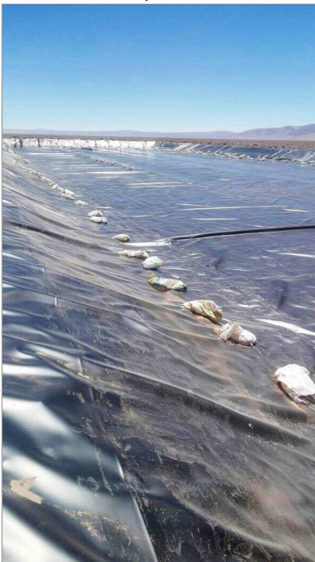
Photo 1. Rincon Lithium Project – Pond construction works; lining installation of Pond 2.
