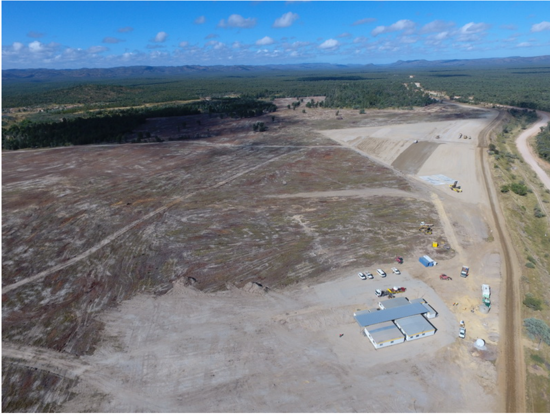
Figure 2: The site compound, laydown area and ongoing site clearing.
