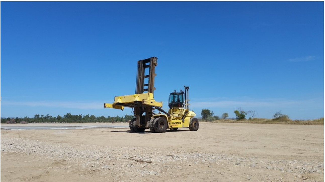
Figure 3: Hardstand/ laydown construction 70% complete.
