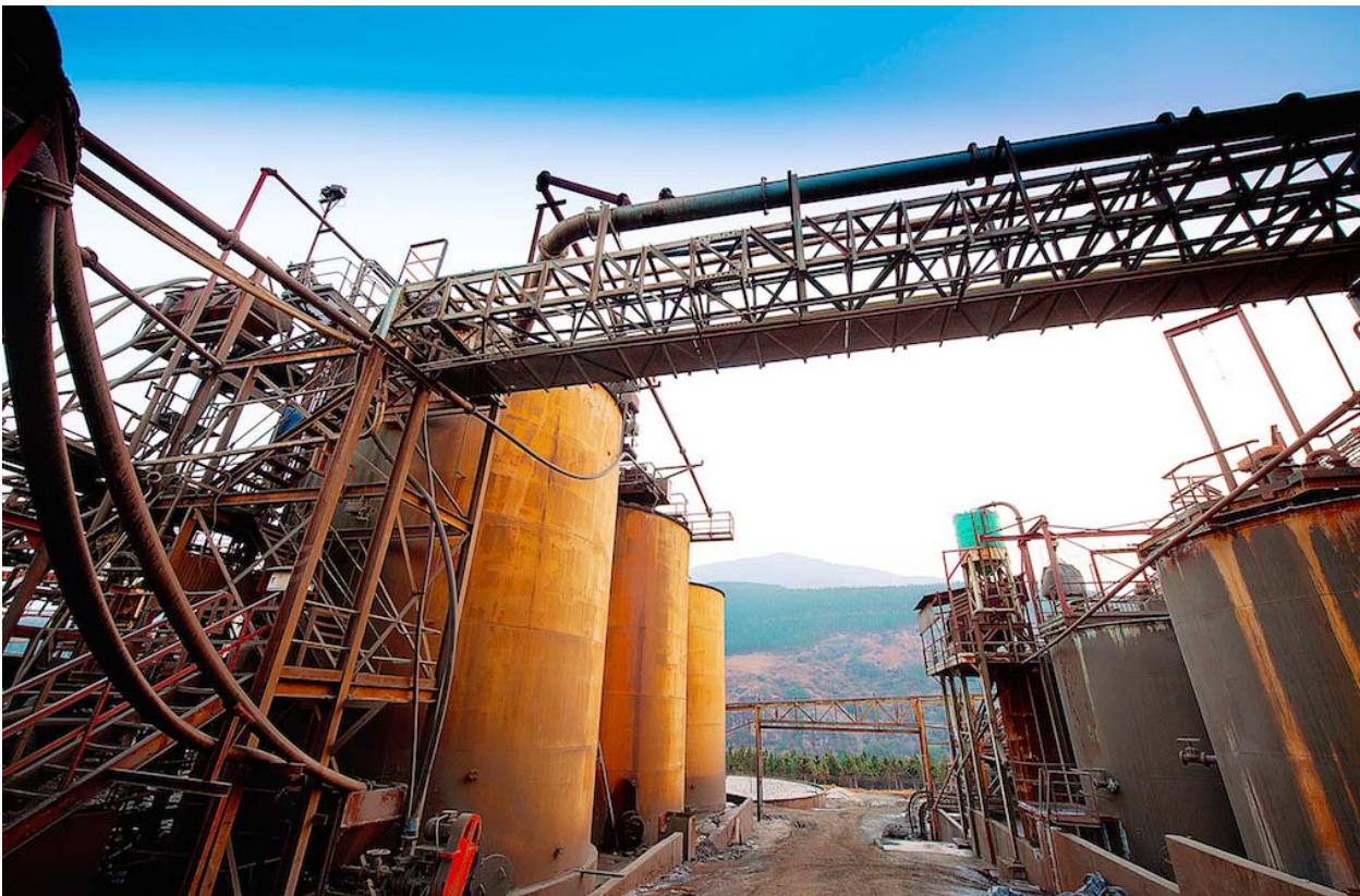
Figure1: Part of TGME plant picture
