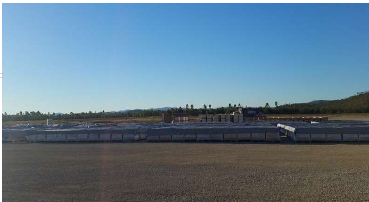
Figure 1: Solar panels stored on laydown area.
