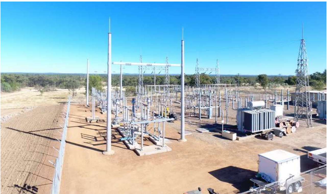
Figure 3: Ergon-Kidston Substation 75% complete.
