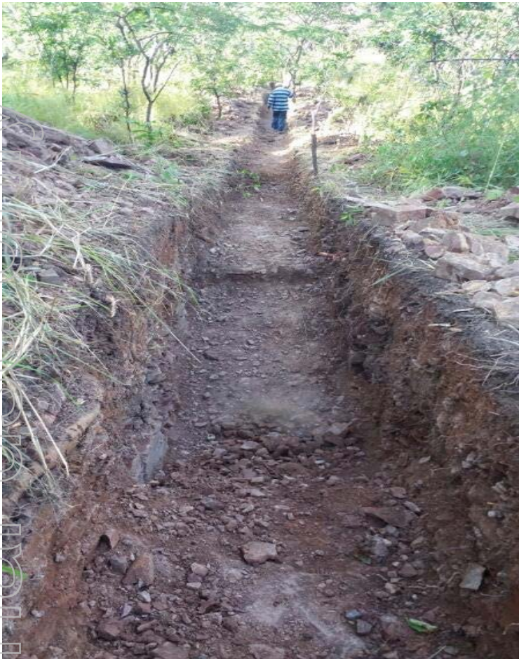
Trenching Work at Mukabe-Kasari
