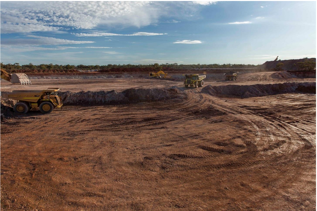
Penny's Find - digging in the hanging wall
