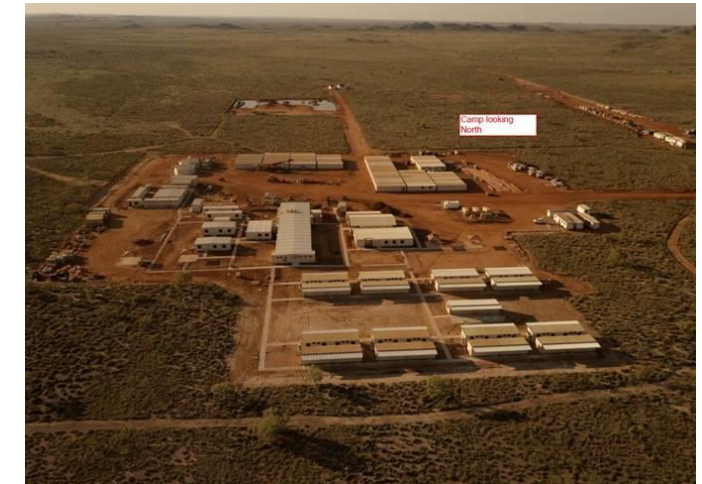
CAMP BUILDING INSTALLATION
