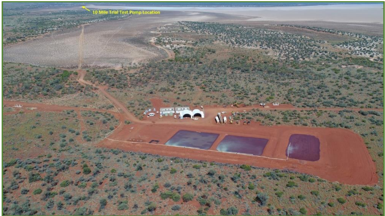
Pond Construction Verification and Leakage Trial Area
