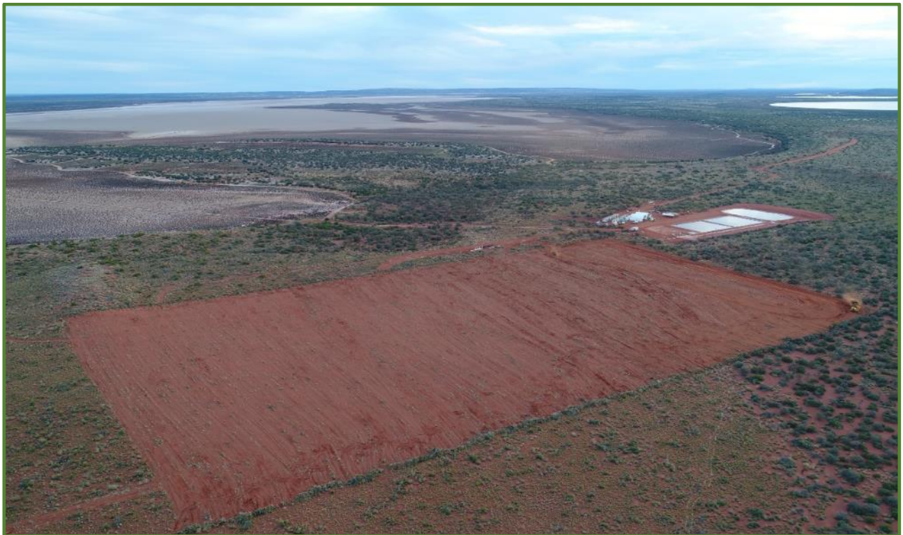
Pilot Pond Area Under Construction
