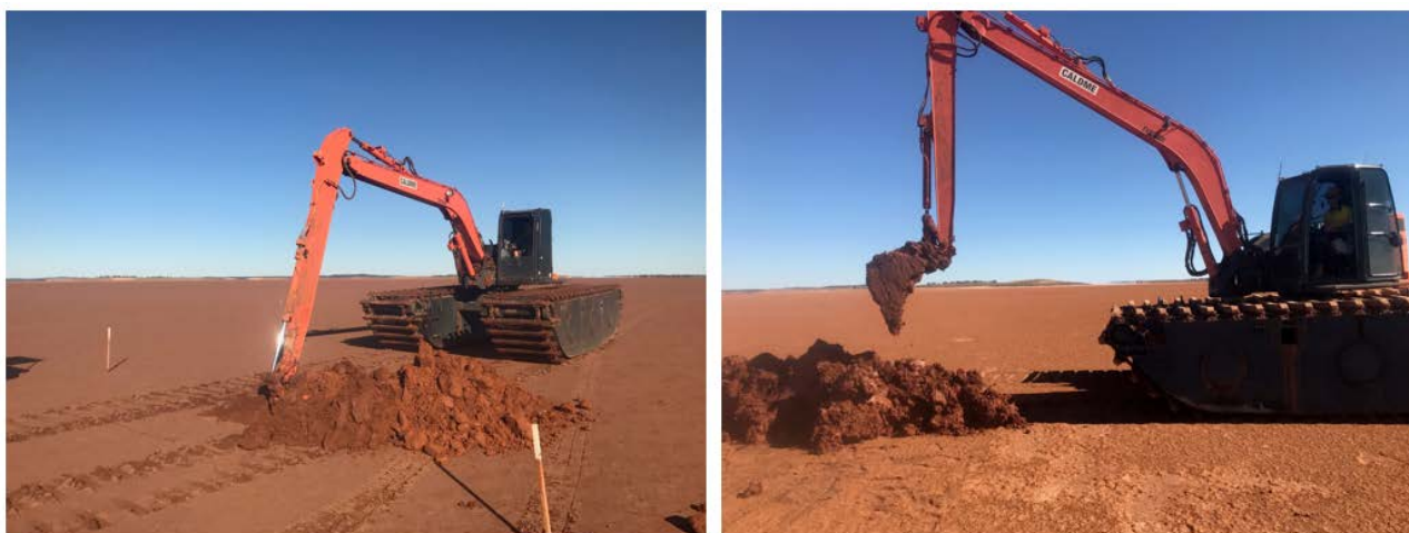
Figure 11: Amphibious Excavator on Lake Ballard
