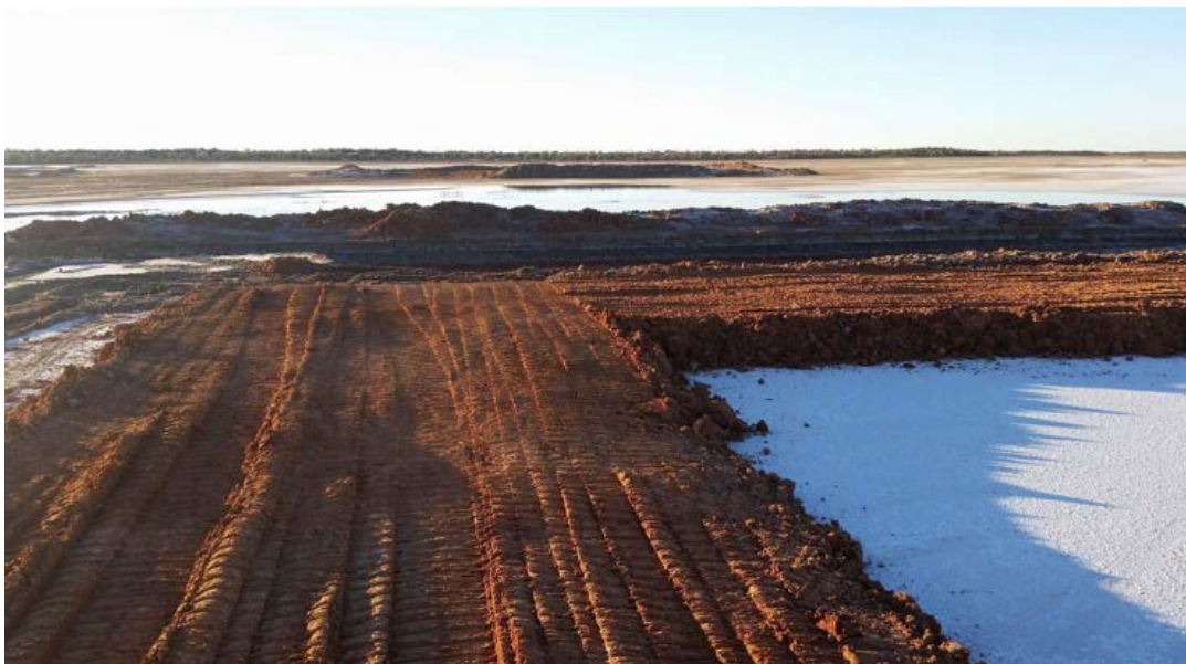
Figure 5: On-lake Evaporation Pond Construction at Lake Wells
