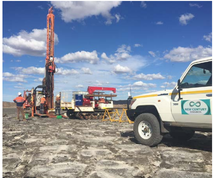
Figure 1: Tailings drilling underway at the Century Zinc Mine
