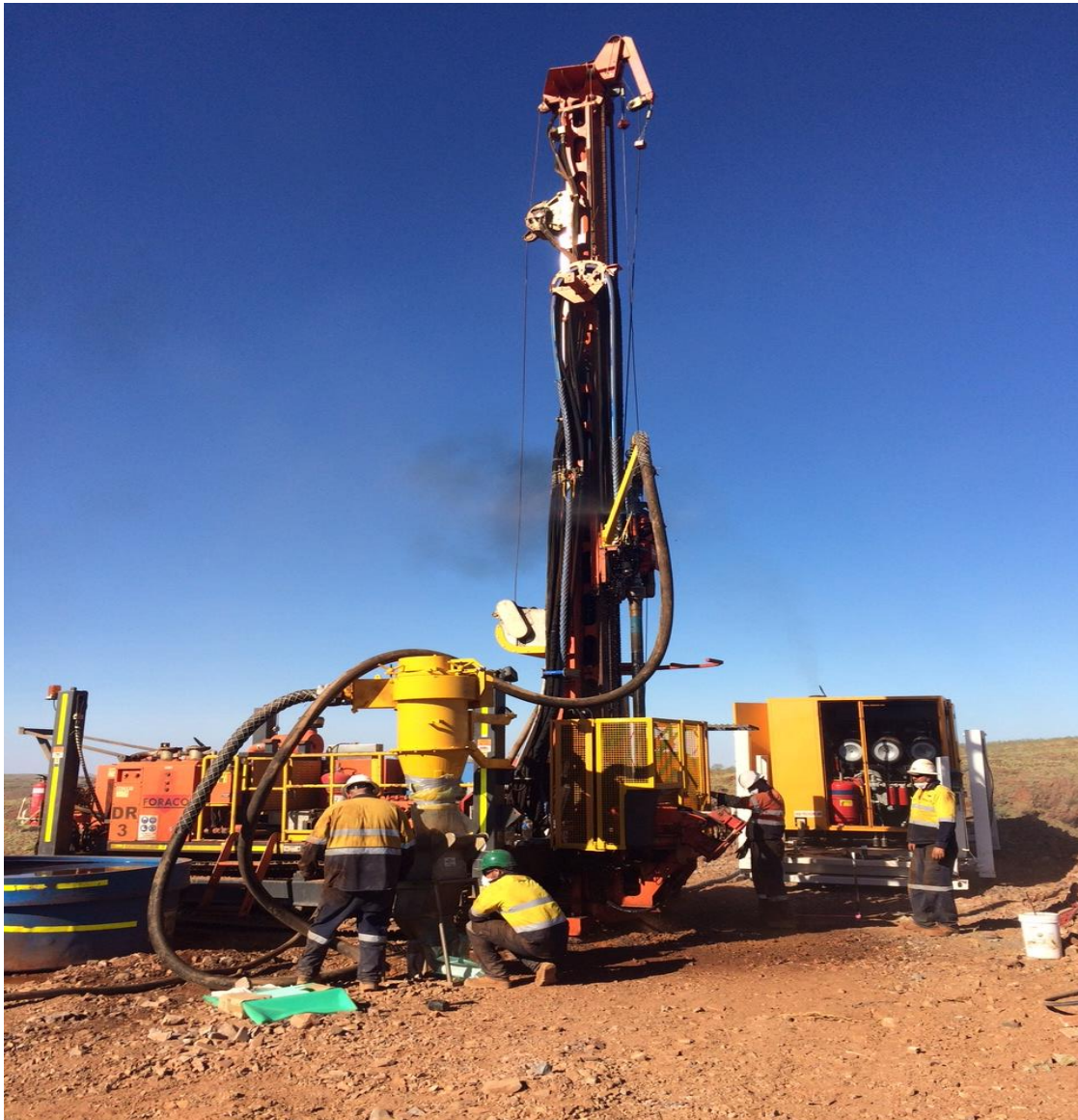
Figure 1: Drill rig on site at Sulphur Springs
