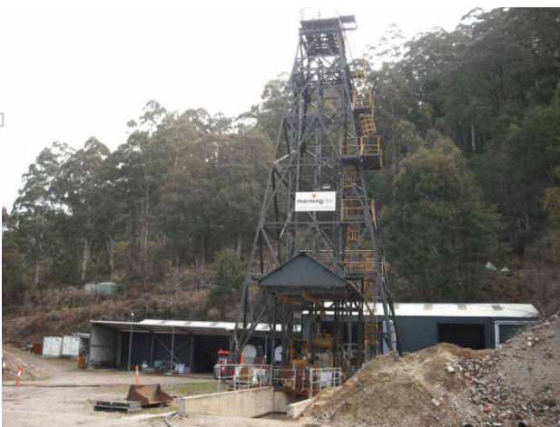
Photo 1 Morning Star Headframe
