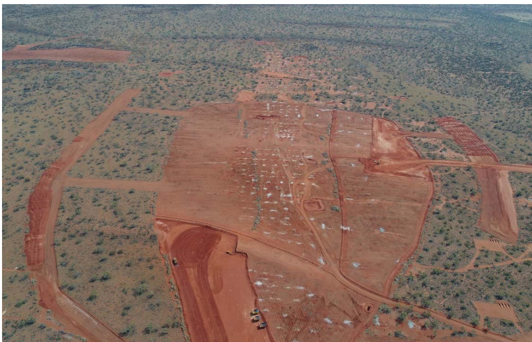
Gruyere Stage 1 pit clearing
