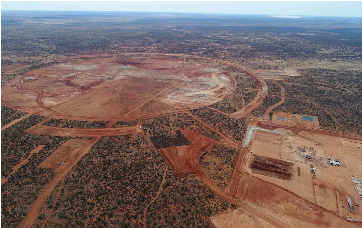
Aerial view of cleared TSF
