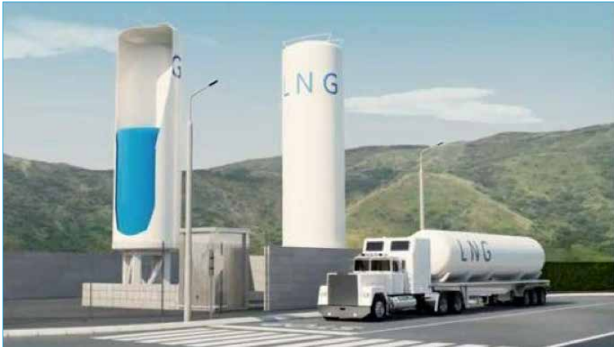
Conceptual virtual pipeline system of (micro) LNG storage and trucking of LNG to end consumers (image courtesy of BHGE).
