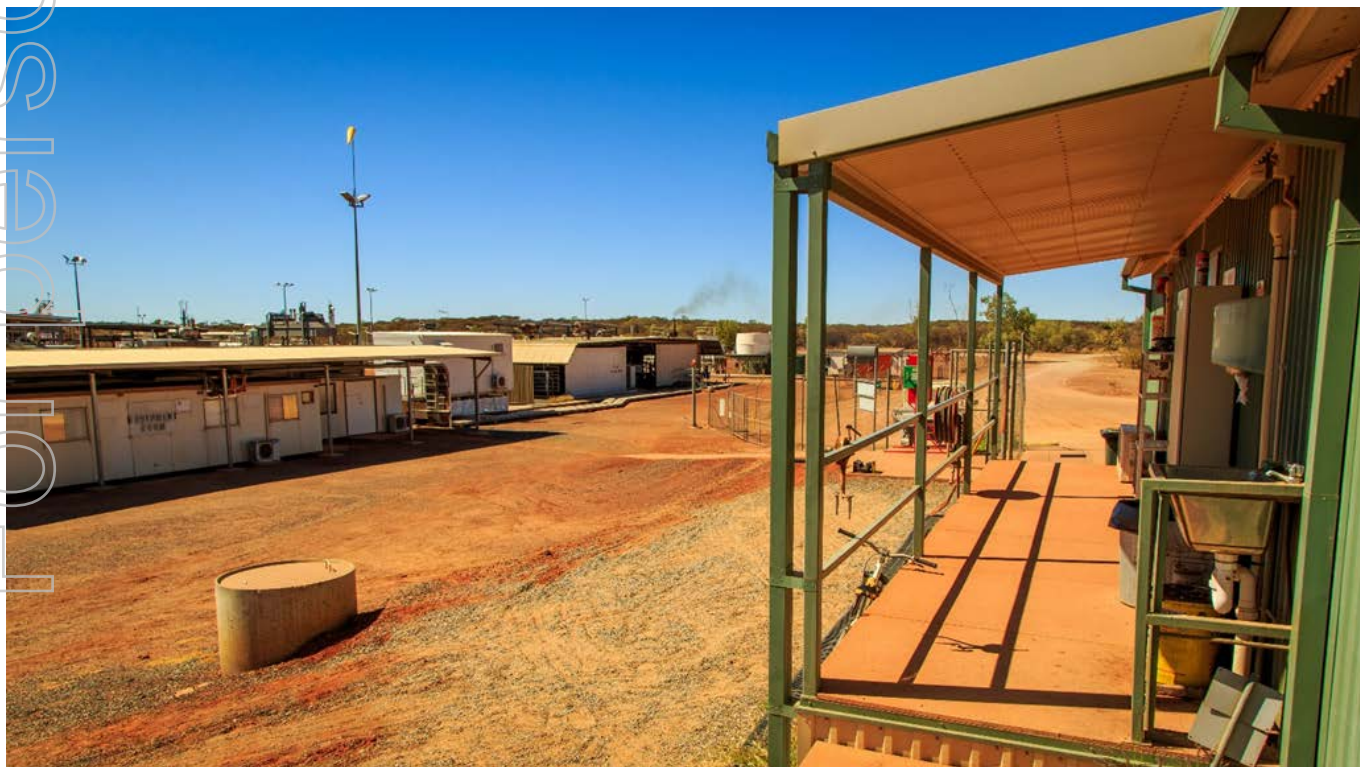
Figure 1: Back of control room at Central Treatment Plant (CTP)
