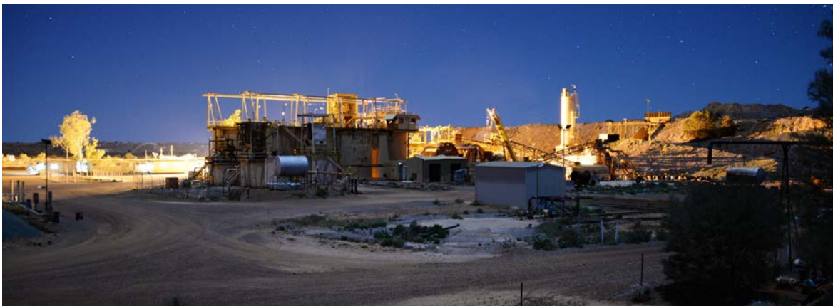
FGP Processing Facility
