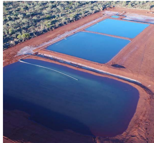
Verification Pond Trials Lined and Unlined
