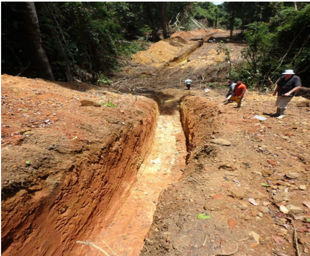
Image 2. Trenching at Turesi
