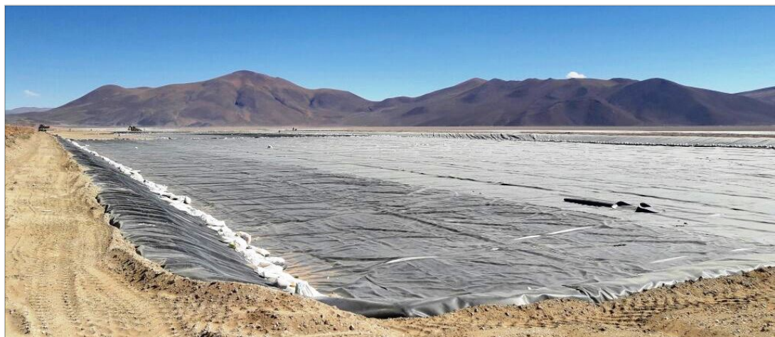
Photo 1. Rincon Lithium Project – Stage 2 Evaporation Ponds, Lining Works
