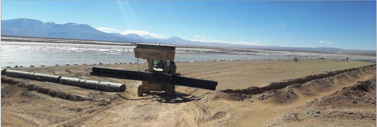
Photo 2. Rincon Lithium Project – Stage 2 Evaporation Ponds, Lining Works
