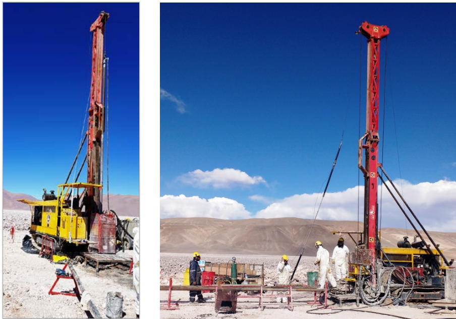
Photos 6 & 7. Rincon Lithium Project – Exploration diamond drilling operations
