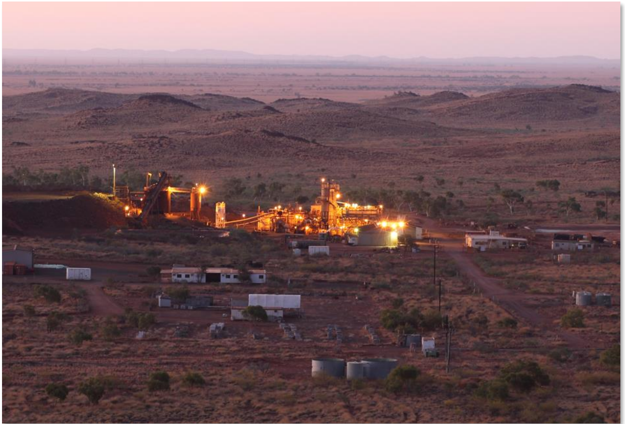
Figure 2: Radio Hill Plant at dusk on Saturday 25 November 2017.
