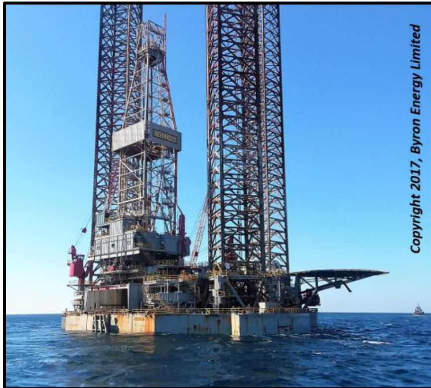
The EnSCO 68 independent leg jack up drilling rig under tow on November 26, 2017 in the Gulf of Mexico
