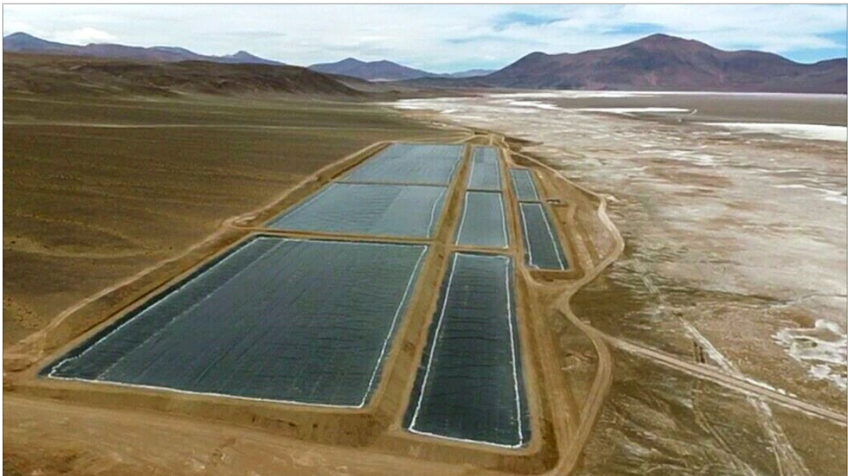
Photos 2 - 3. Rincon Lithium Project – initial Stage 2 Evaporation Ponds
