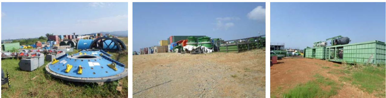
Figure 7, 8 and 9: Mechanical plant and equipment at the Project site contained within 115 sea containers
