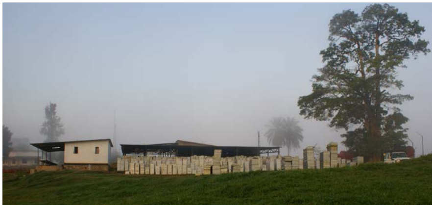
Figure 6: Drilling core sheds at the Project operations camp site.
