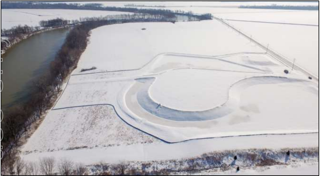
Completed Site Excavation at the Poplar Grove Mine Barge Load-out Facility
