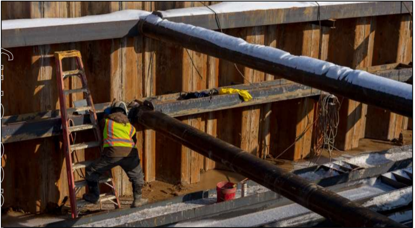
Construction of the Slope Portal to Access Underground Coal
