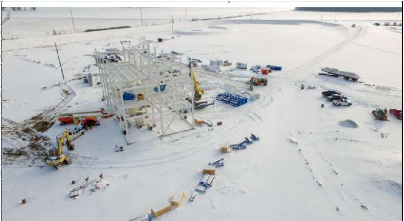
Installation of Internal Coal Processing Infrastructure at the Preparation Plant
