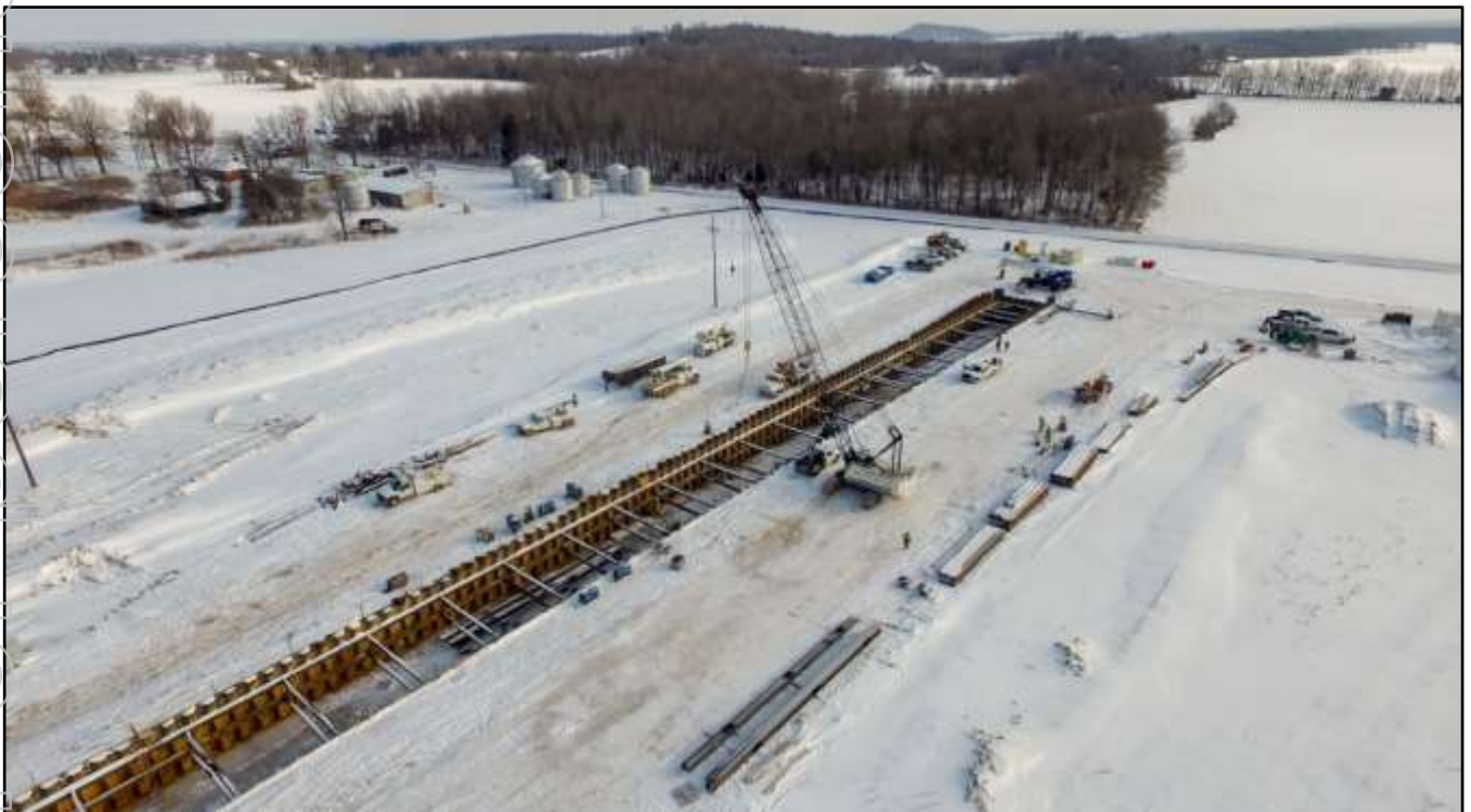
Excavation of the Slope Decline to Access Underground Coal
