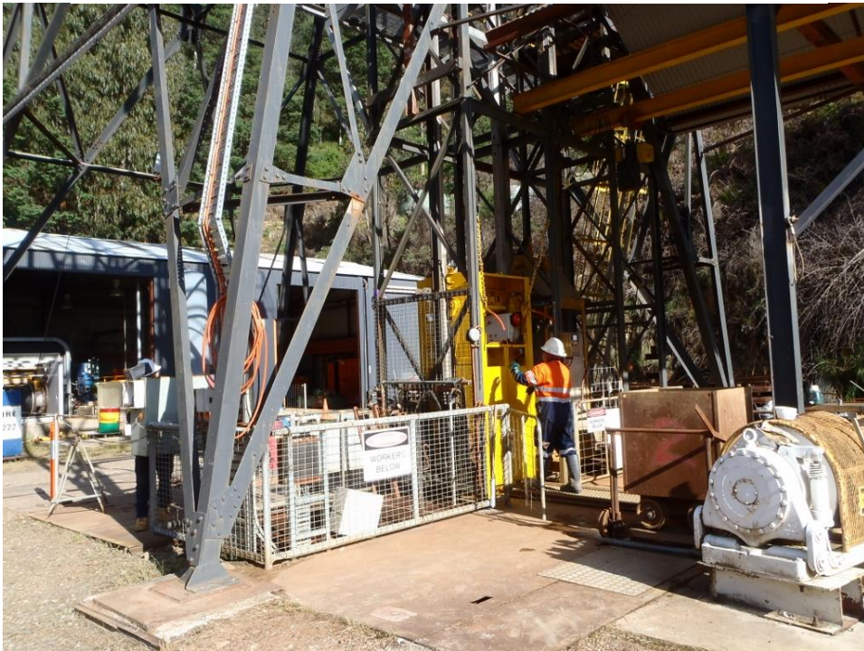
Figure 1. Ore cart being loaded into recommissioned mine cage and shaft
