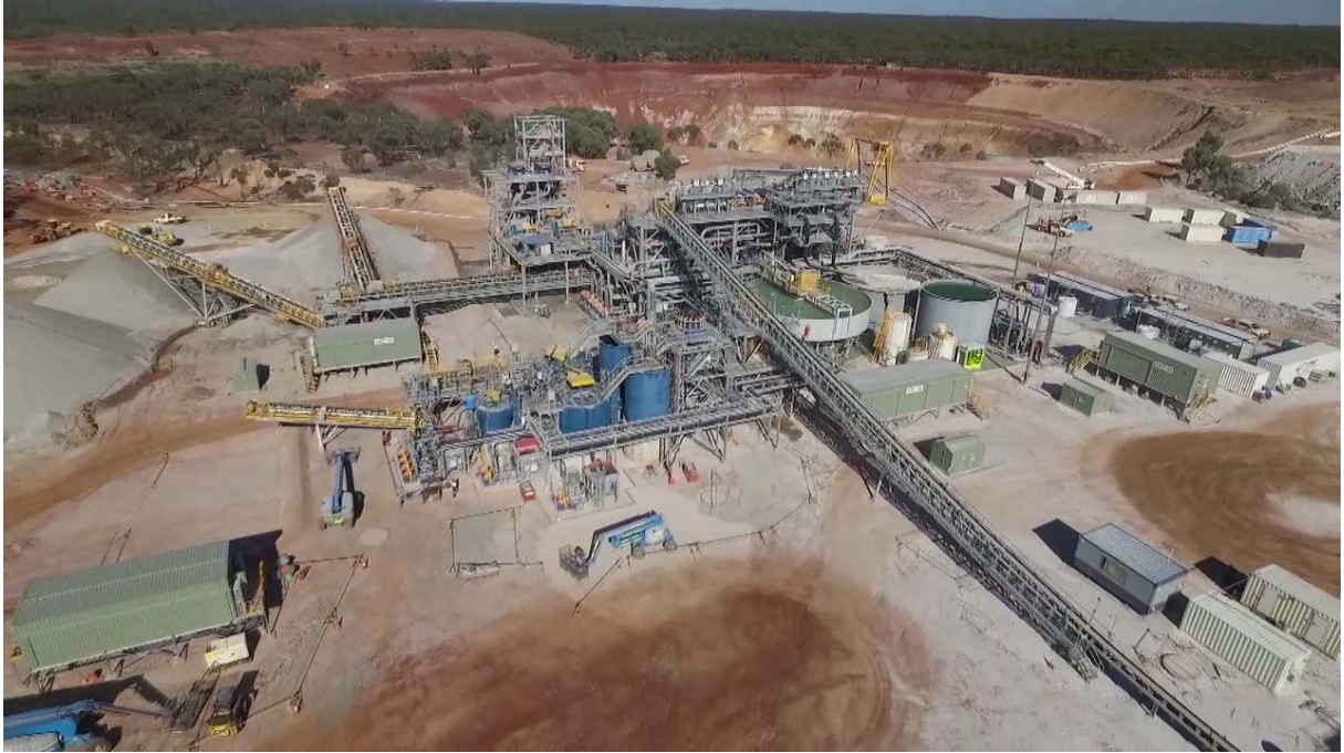
Image 1: Aerial View of Mt Marion Lithium Operation's Processing and Tailings Storage Facilities
