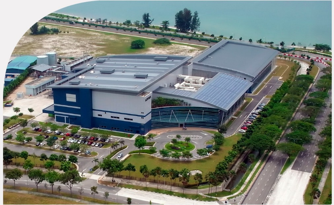
Lonza contract manufacturing facility in Singapore
