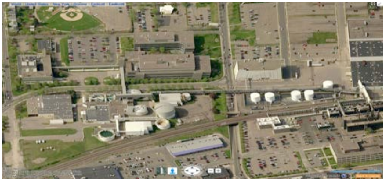
Figure 1 – Huron Campus, the proposed location of the Imperium3 New York lithium-ion battery plant
