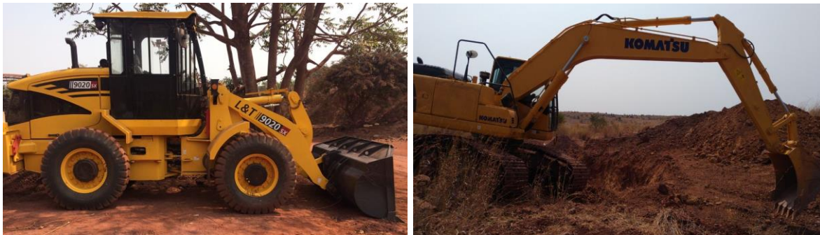
Part of new fleet on site and operating
