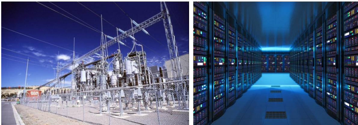
(Picture (Left) Actual photo of Hunter Energy (Right) example of Data Centre)
