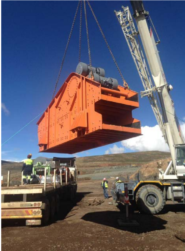
DMS components being offloaded on site at Mothae
