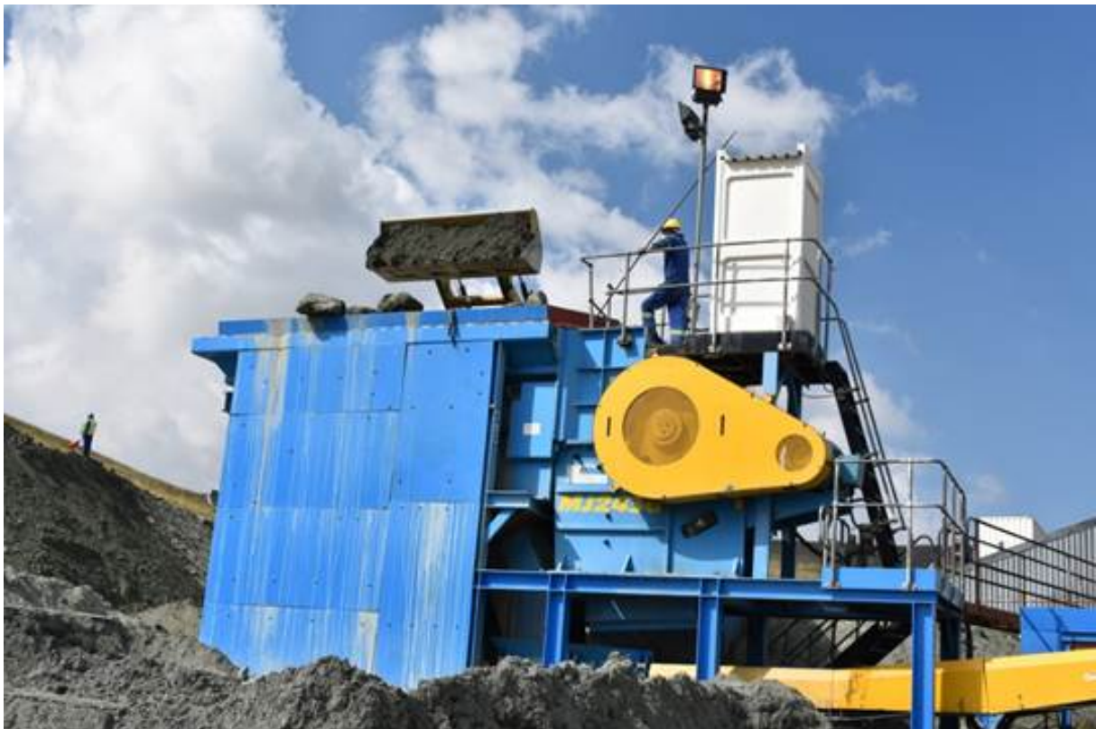
Primary crusher of the re-commissioned bulk sampling plant at Mothae
