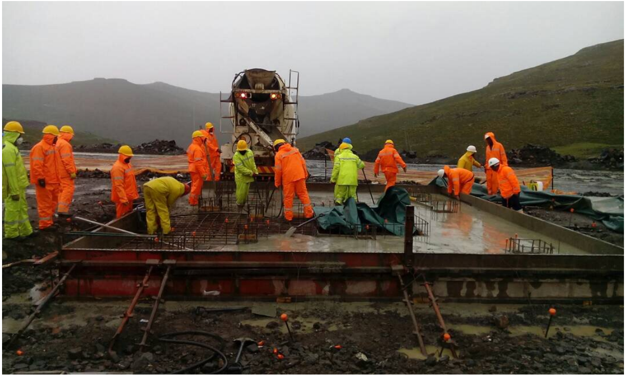
Site works/ civils for the new 150 tph Mothae diamond plant
