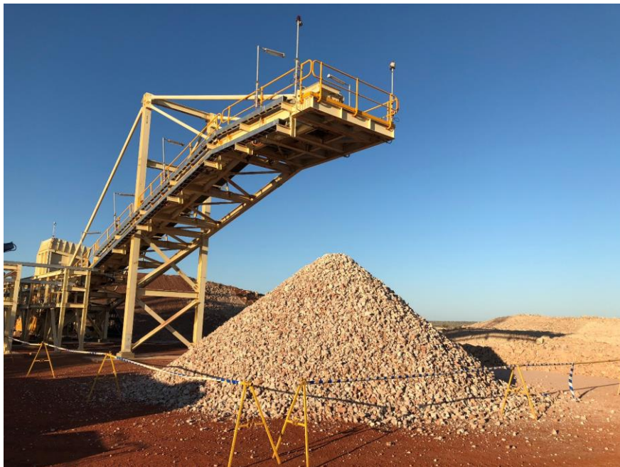
Close-up – crushed ore stockpile from commissioning
