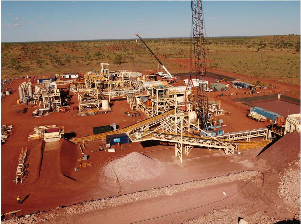
Crushing system commissioned
