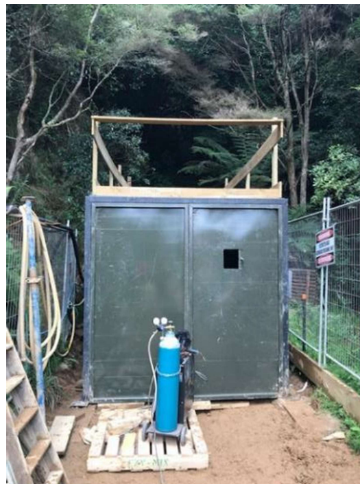
Figure 2 - Completed ventilation lock at No 8 Level Portal
