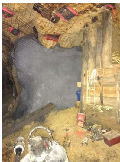
Figure 4- completed ventilation seal in the No 8 Level drive.
