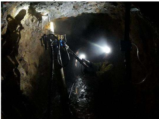
Figure 3 - installation of rock bolts in Keillors Crosscut
