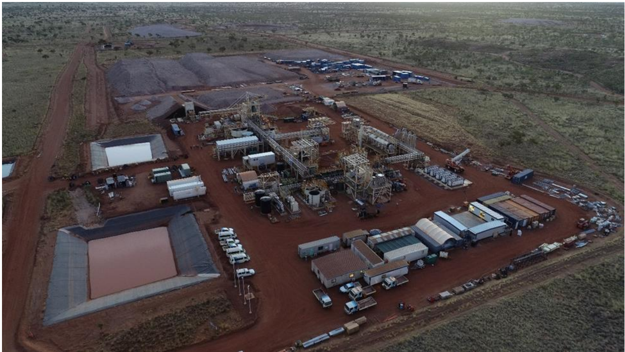
Process plant overview – 21 May
