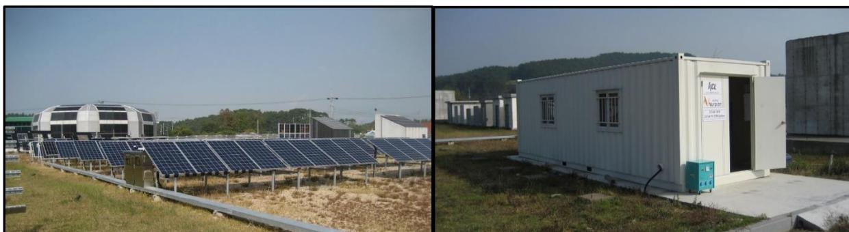
**Figure 1: 20kW solar PV integrated with two 25kW V-KOR battery and the electricity grid in a field test site at Seosan-si in Korea.**
