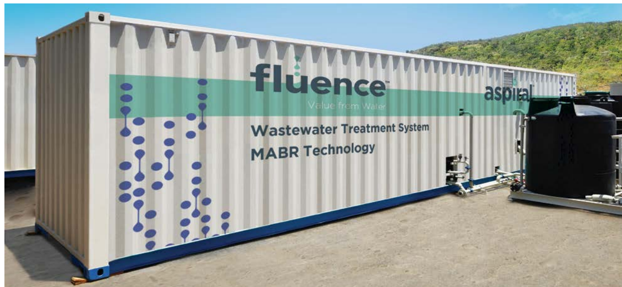
Aspiral™ was chosen for this project in part due to its small footprint and ability to reliably achieve Class 1A effluent.
