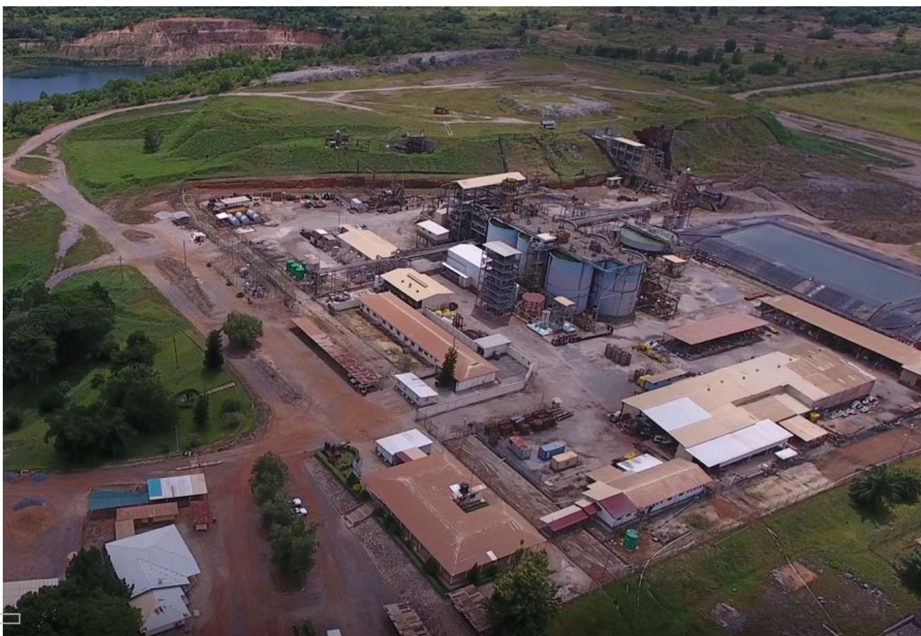
Figure 1: Bibiani Gold Mine and Processing Plant
