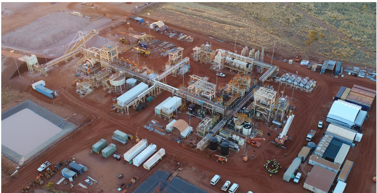
Process plant overview – 17 July 2018
