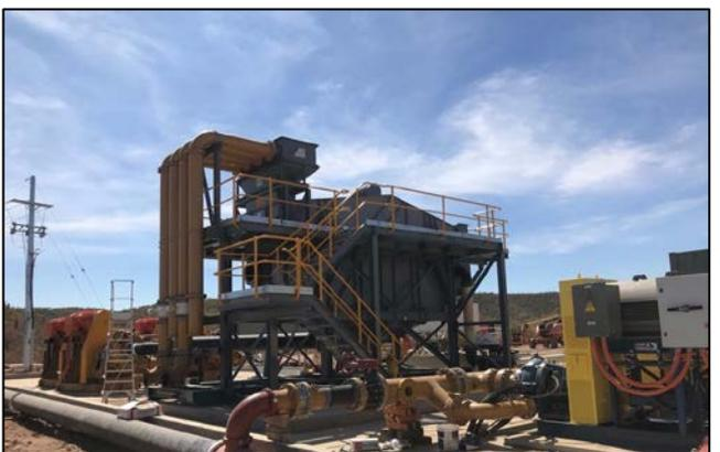
Figures 6 & 7: Water Storage Tank construction complete (left) and installation of the Slurry Feed Hopper (right)
