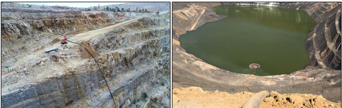
Figures 12 & 13: Installation and commissioning of the Tailings Deposition Line into the historical open pit
