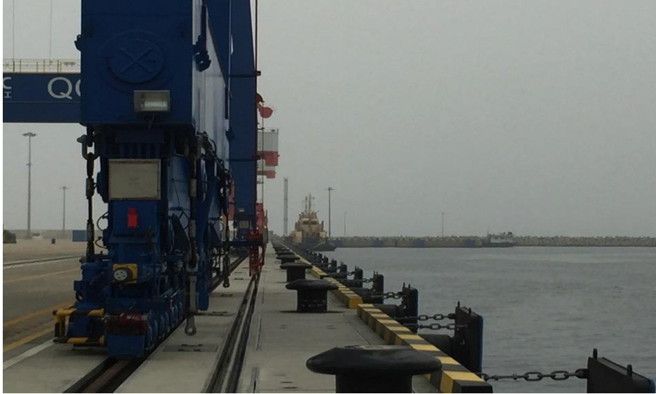
Figure 4: The wharf and ship berthing area of the Kribi Deep Sea Port
