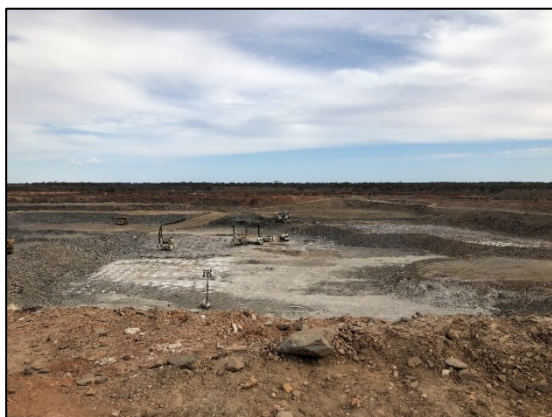
Blast hole drilling
