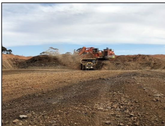
Mining excavations to provide additional sump capacity
