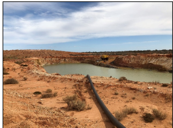
Water re-circulation via historical pits and lines
