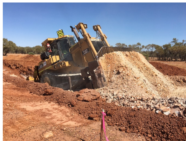
CAPTION: D9 dozer undertaking trial stripping of share overburden at Ardmore.
