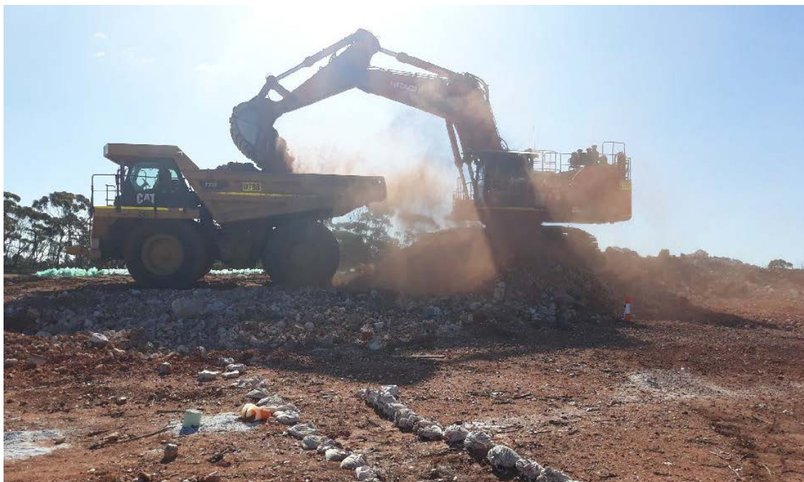
Figure 1: Extraction of overburden at the Sinclair Caesium Mine is underway
